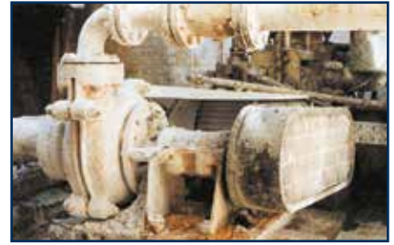
AESSEAL® installed seal on a paper stock pump
